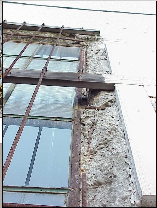
Frye Industrial Buildings Spalling Concrete at Window Jambs and Heads. This Damage Was Caused by a Combination of Rebar Too Close to the Edge of the Jamb and Corrosion of the Embedded Steel Window Frames.
